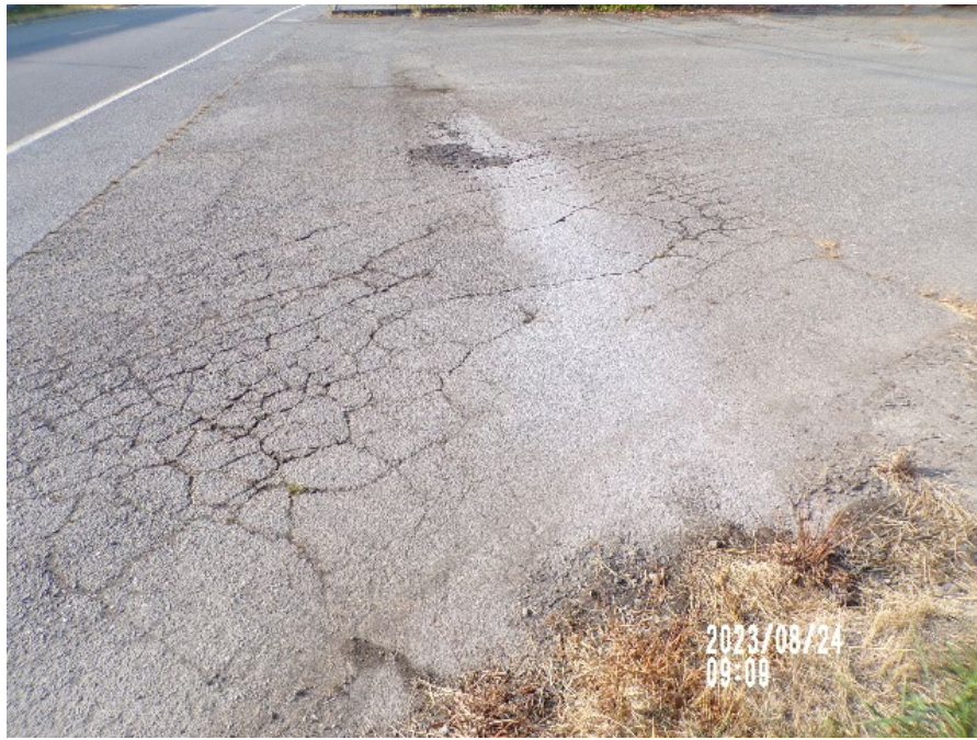
Photograph 3. August 2023 View facing south, alligating on east side of OU1
