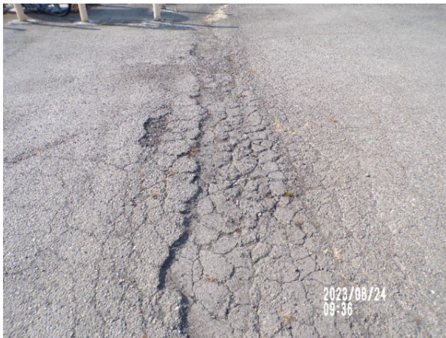
Photograph 6. View facing south, alligating at OU1 Area 22 near 4th Street parking area. August 2023
